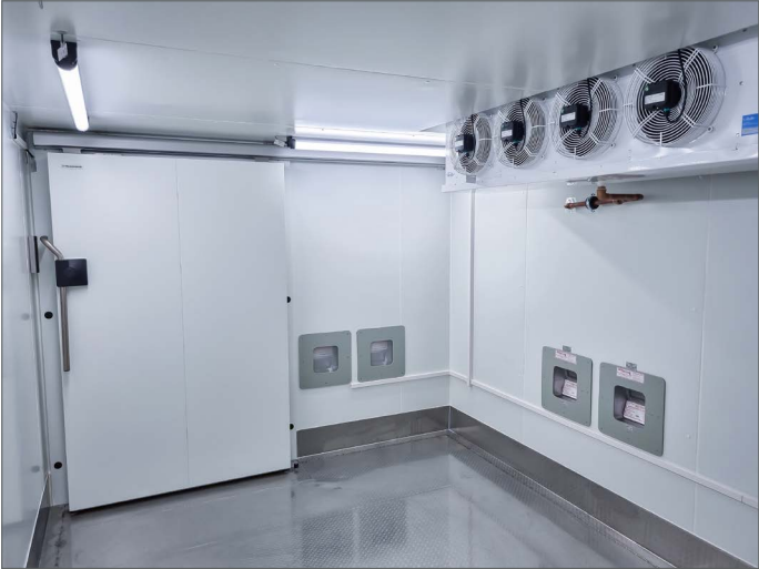
Lock with active -20 \text{ }^\circ\text{C} cooling
