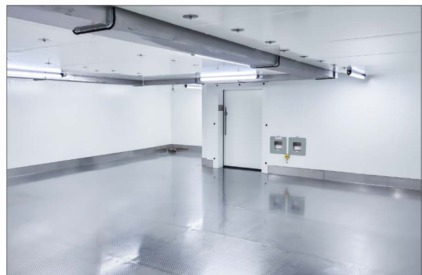
185 m 3 storage room with flexible temperature control from -20 °C to -90 °C
